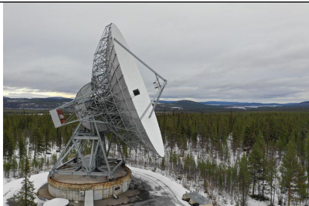
The EISCAT Kiruna site antenna. Location: 67°51'38"N 20°26'07"E EISCAT Kiruna Mottagarstation SE-981 92 Kiruna Sweden
