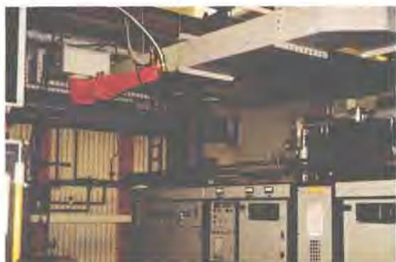
This photo shows one transmitter amplifier (125 kW), a waveguide part and a dummy load.
