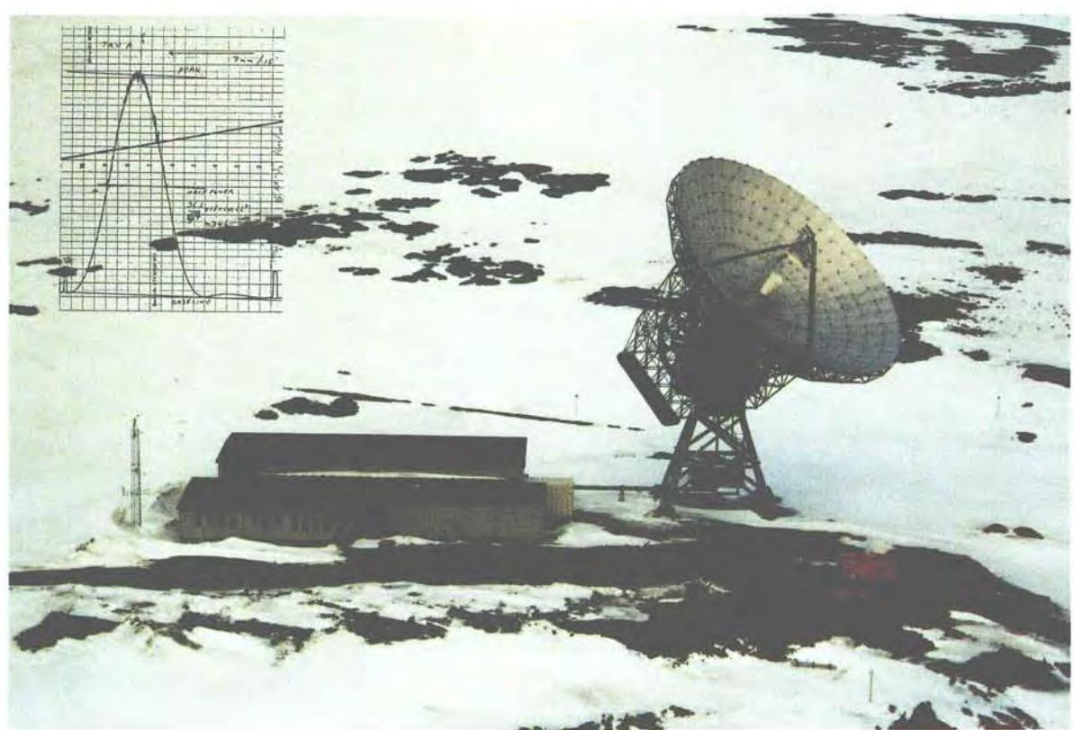
The ESR antenna after erection in September 1994 (upper photo) with the view towards the NW along Adventdalen. The lower photo shows the antenna and site building after completion. The insert shows the main lobe of the antenna pattern measured with Taurus-A drift scan.
