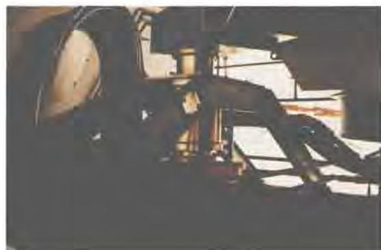
The waveguide extends from the final combiner in the transmitter hall up to the antenna, where the power passes the azimuth (photo) and elevation rotary joint.
