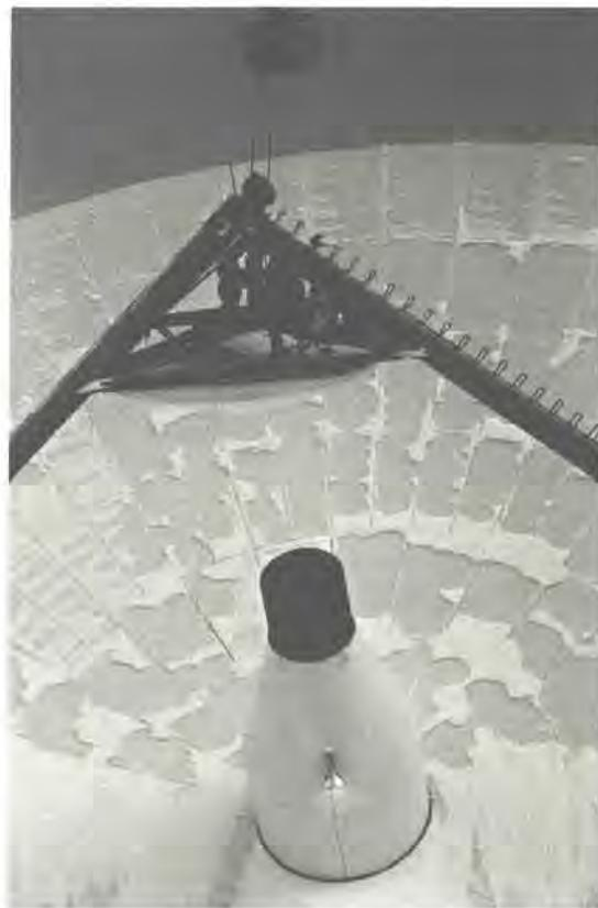
The regular quadri-annual bolt tightening of the UHF antennas took place at all sites in 1995. Events which caused shorter, but not critical, UHF operation interruptions were the repairs of an elevation motor, rail undercast, pintle bearing, fixing of leakages in the foundation roof, and elevation rotary joint restoration.
