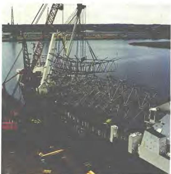
On-site construction of antenna reflector support structures. The feed horn is seen in the centre.
